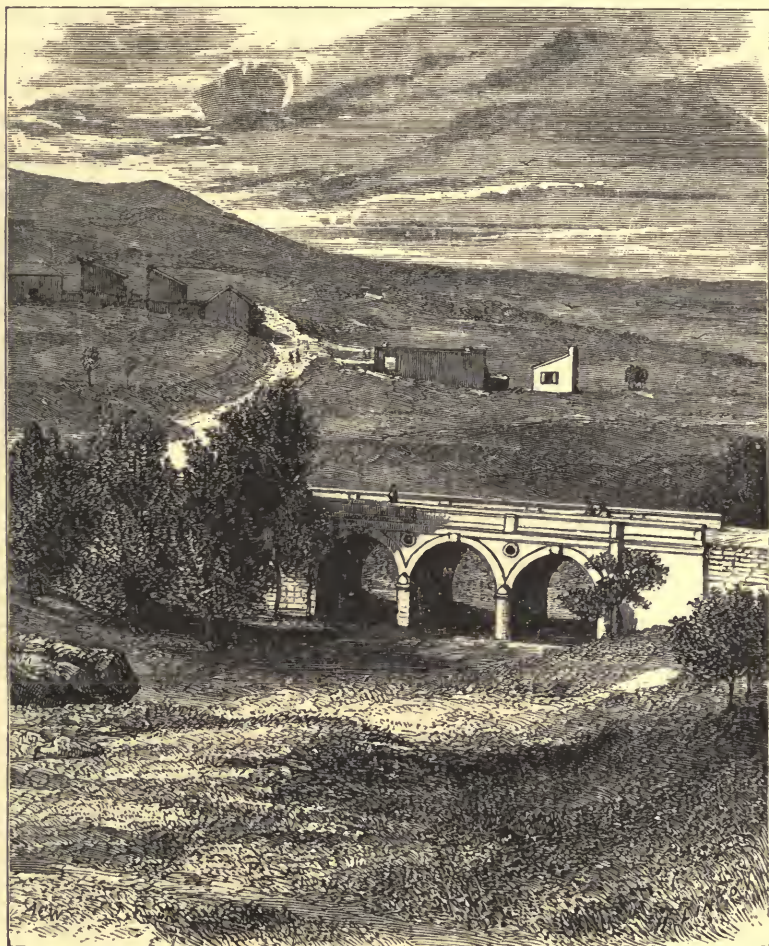
BRIDGE AT ELEUSIS.
